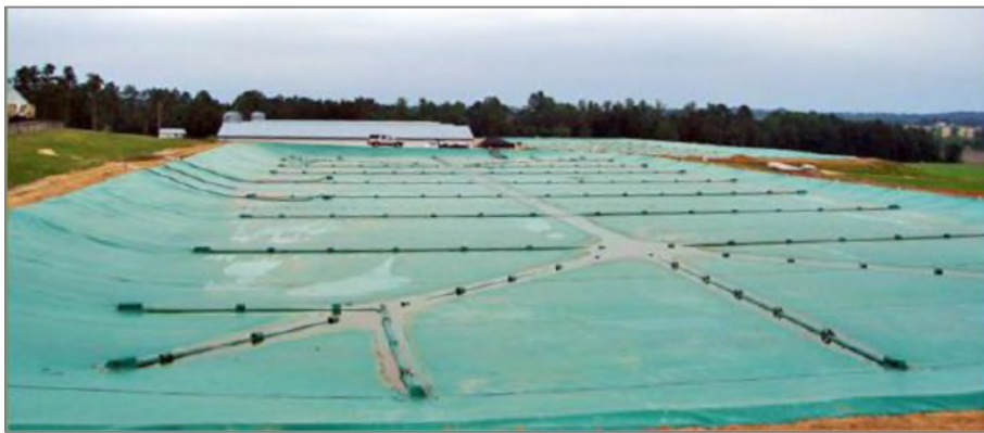
Figure 2: Covered Lagoon Style Digester Prior to Gas Production
