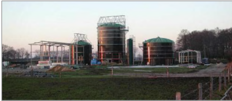
Figure 3: Complete Mix Anaerobic Digester
